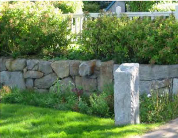
Authentic materials used with dry stack method to appear native to site
