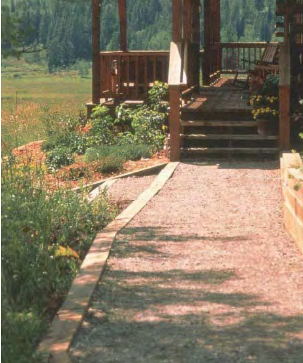
Wood header is combined with pervious crushed rock surface to define path
