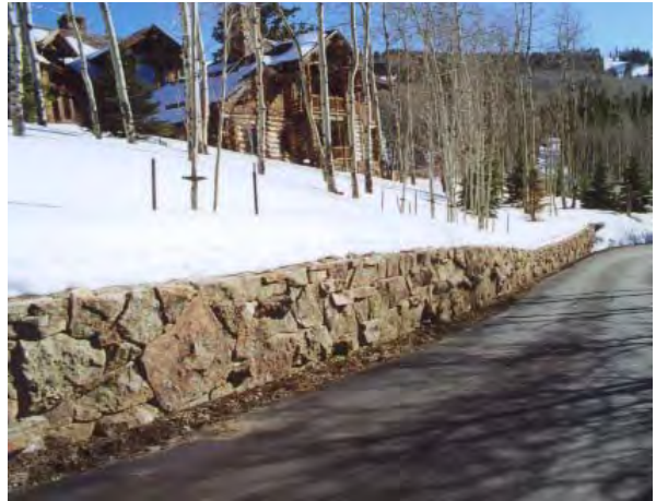
Retaining wall minimizes site disturbance and transitions naturally into existing landforms
